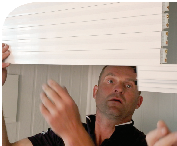
Installing the interlocking curtain
