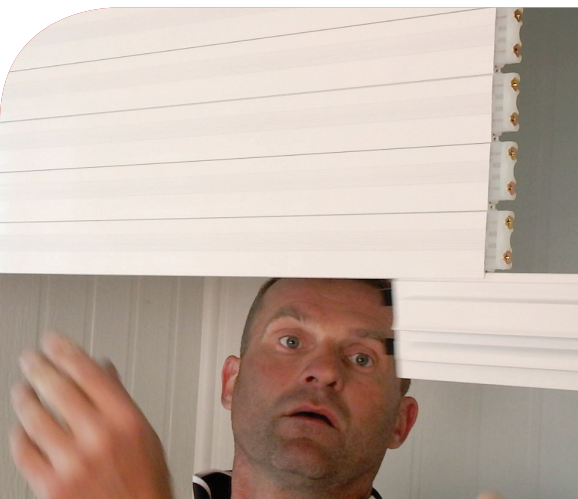
Installing the interlocking curtain
